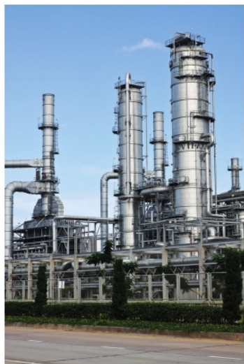
▲ fig B Several different processes take place in oil refineries. This distillation plant is just one small part of a large refinery.
