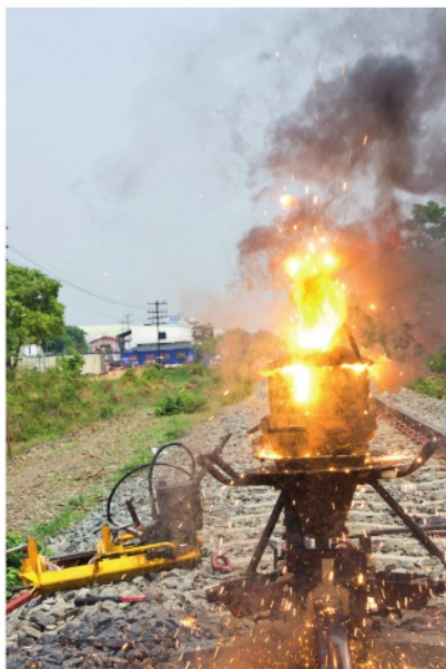
fig B The thermite reaction. The flame comes from the highly exothermic reaction forming molten iron. The molten iron will be used to fill the gap between two rails and form a strong join between them.
