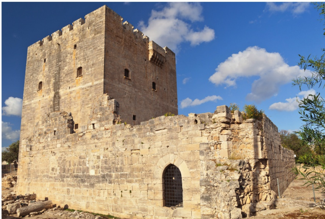
▲ fig A Many old buildings are made from carbonates such as limestone. Centuries of reaction between limestone and acids in the atmosphere have caused damage to the walls of Kolossi Castle in Cyprus.
